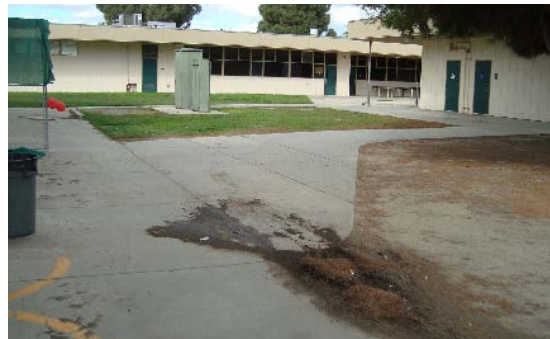
Poor concrete/asphalt conditions campus wide.
