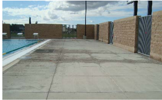
Pool in need of modernization; deck resurfacing.
